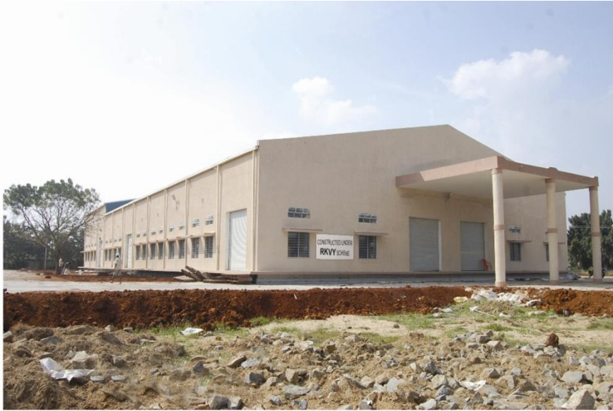
NEW GODOWN CONSTRUCTED AT A.P.S.S.D.C.LTD., SRIKALAHASTHI UNDER R.K.V.Y. SCHEME
