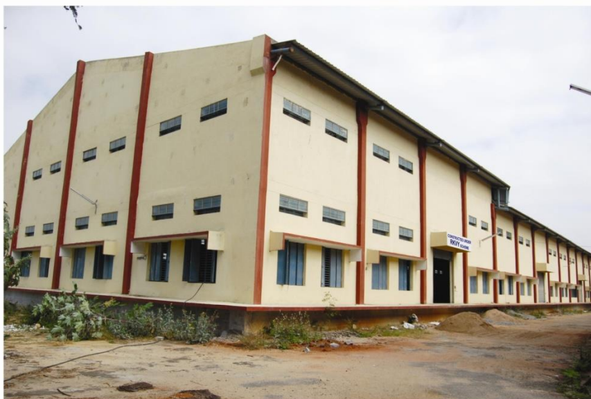
NEW GODOWN CONSTRUCTED AT A.P.S.S.D.C.LTD., WARANGAL UNDER R.K.V.Y. SCHEME
